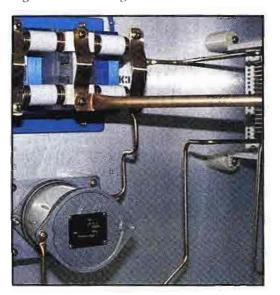
Inspect AM system antenna tuning units for loose connections or contaminants that could cause arcing.
