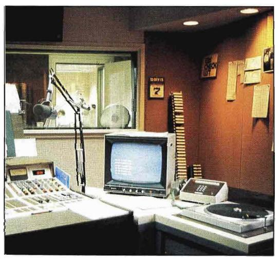
Control room lighting must illuminate the work surfaces (console) as well as other controls. If a CRT is located within the work area, it must not reflect glare from the lighting source.
